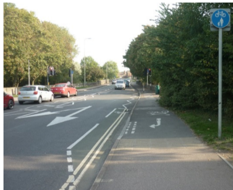
Figure 3-6 Inconsistent provision for cyclists on Drayton Road
