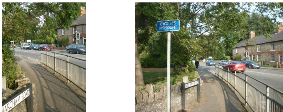
Figure 3-8 Pinch point on the southwestern corner of Drayton Road and Marcham Road
